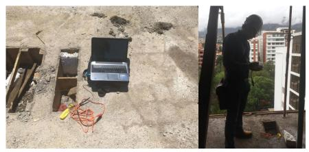
Figure 8: Slab Maturity Index Readings.
